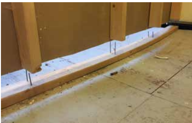
Photos show how far the floor has sagged: detaching from pony walls built only a few years ago and below bottom edge of sheetrock...
