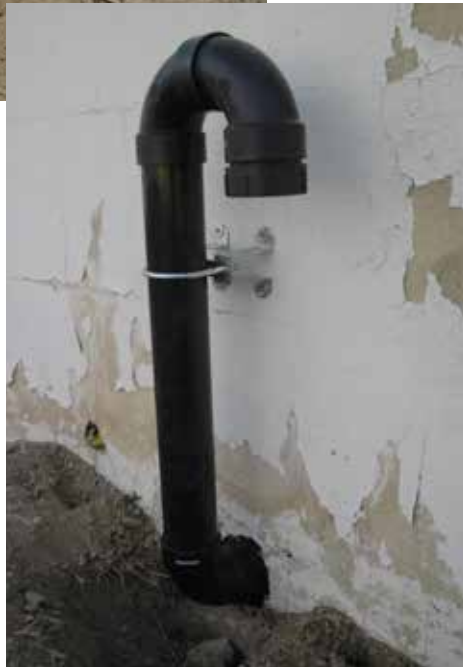
Exterior work: drainage system, venting to foundation,
