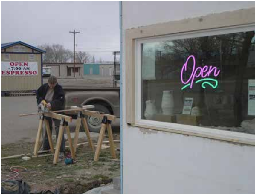
Exterior work: trim, off street parking, signage, landscaping
