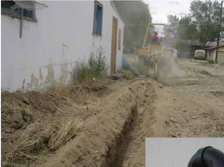
Exterior work: drainage system, venting to foundation,
