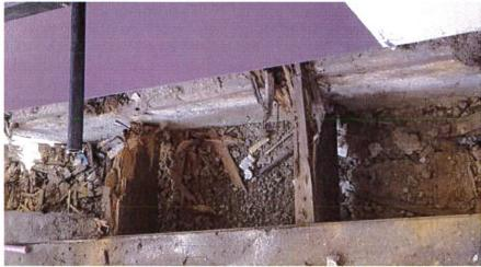
Photos show the complete rotting of original flooring and floor joists. The only thing holding the floor up is the plywood sub-flooring nailed to the original tongue and groove floor... not a stable situation.
