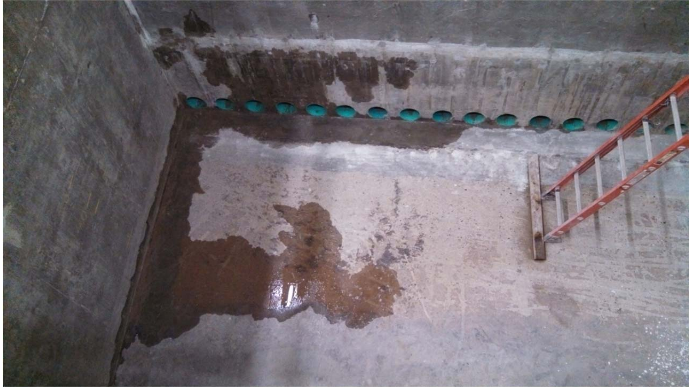
Figure 1. Pix taken by AI V 4/29/2014 w. 8 feet of water in F4. Shows influence on leaks in Cold seam # 1 of F3
