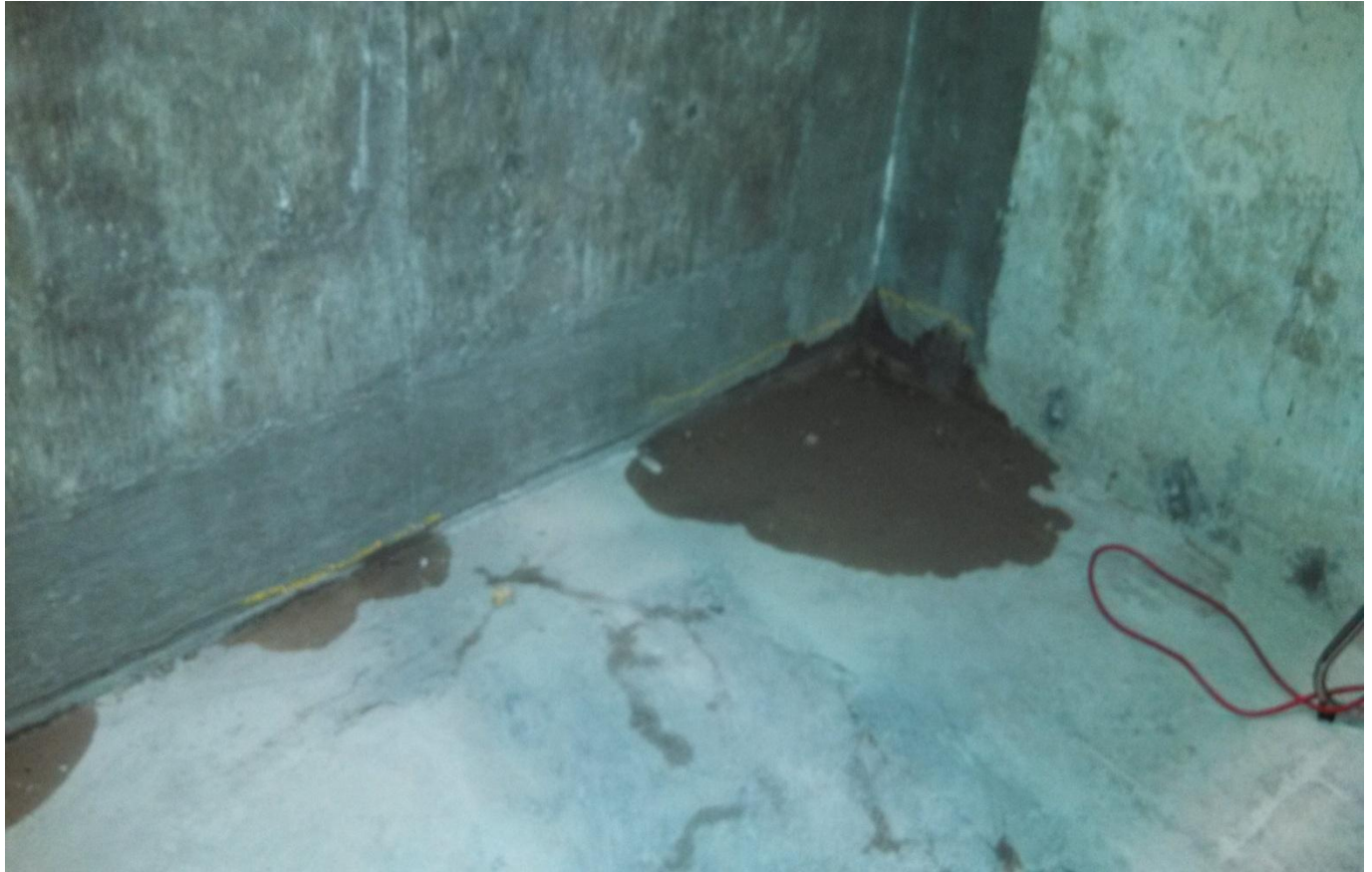
Filter #4 west wall and northwest corner.
