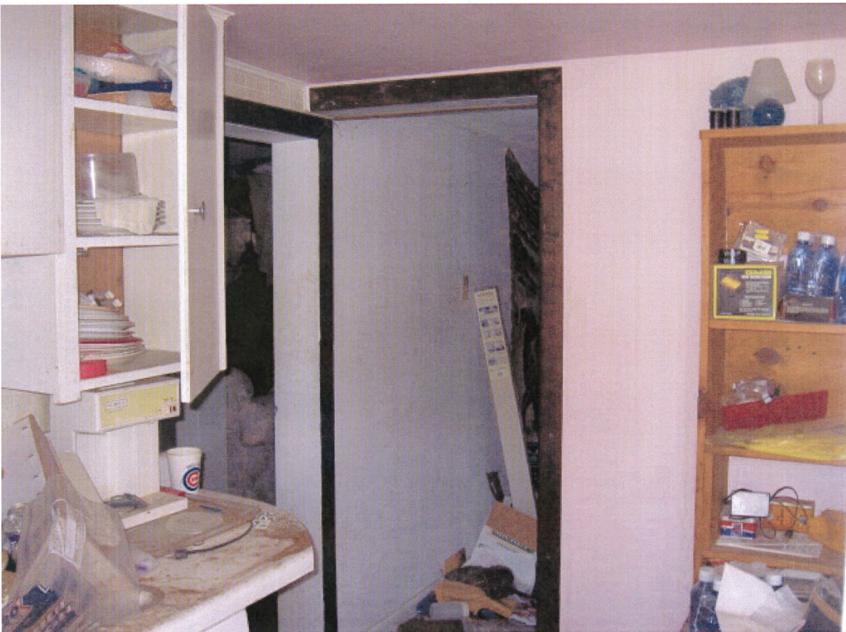
Figure 7. Interior damage and clutter
