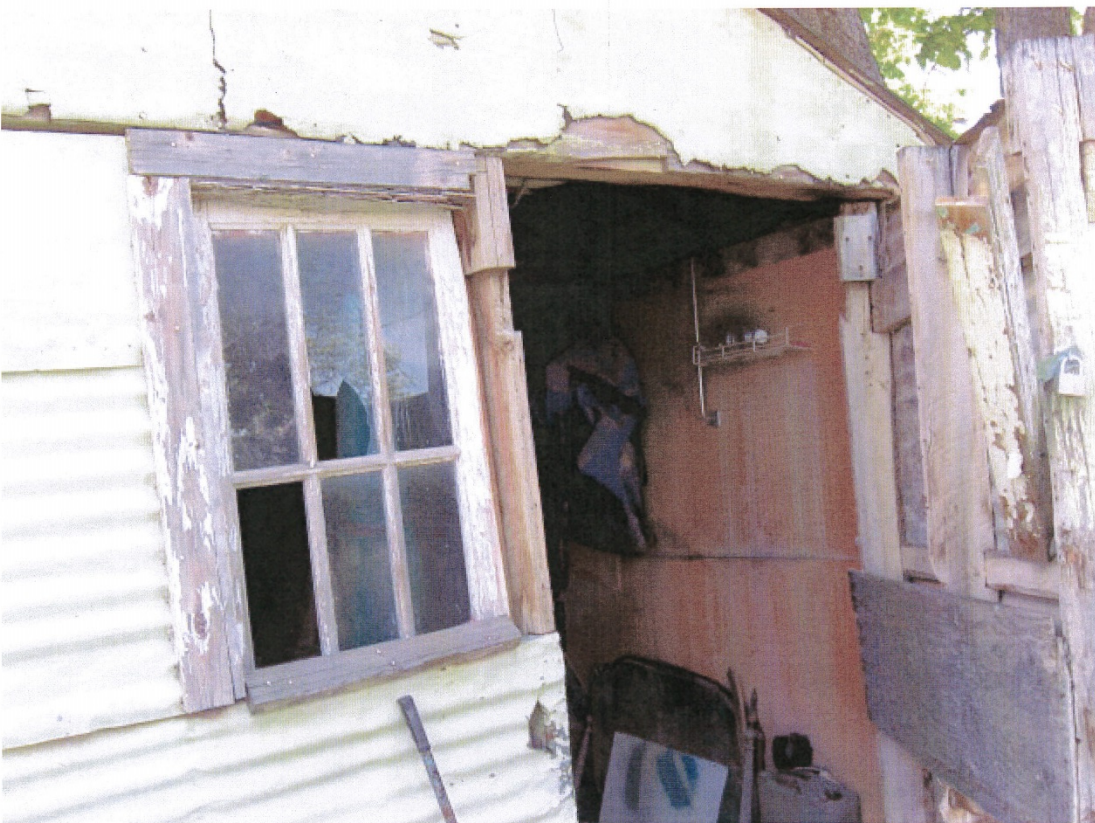
Figure 11. Doorway to shed in Southeast corner of property
