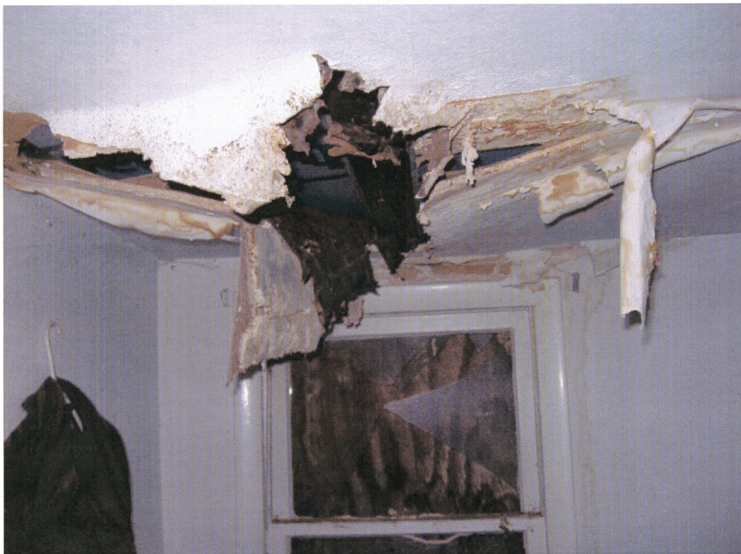
Figure 8. More interior damage and clutter
