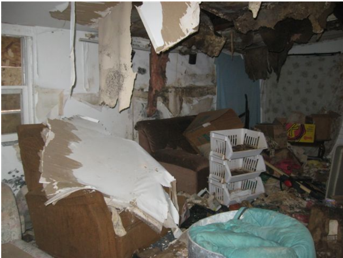
Figure 6. More interior pictures showing ceiling damage
