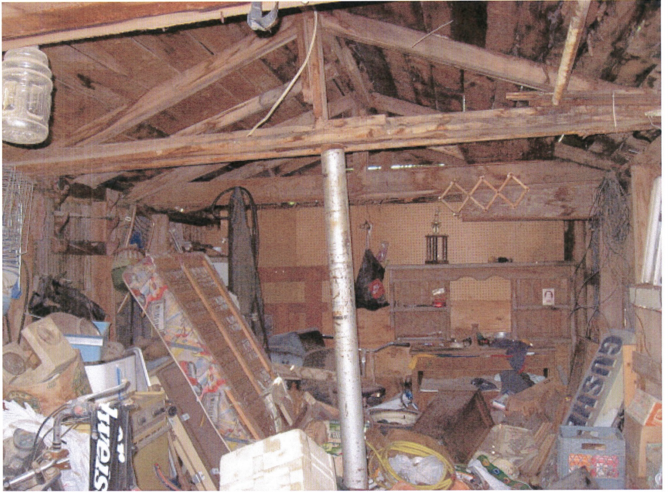
Figure 12. Shed damage and clutter
