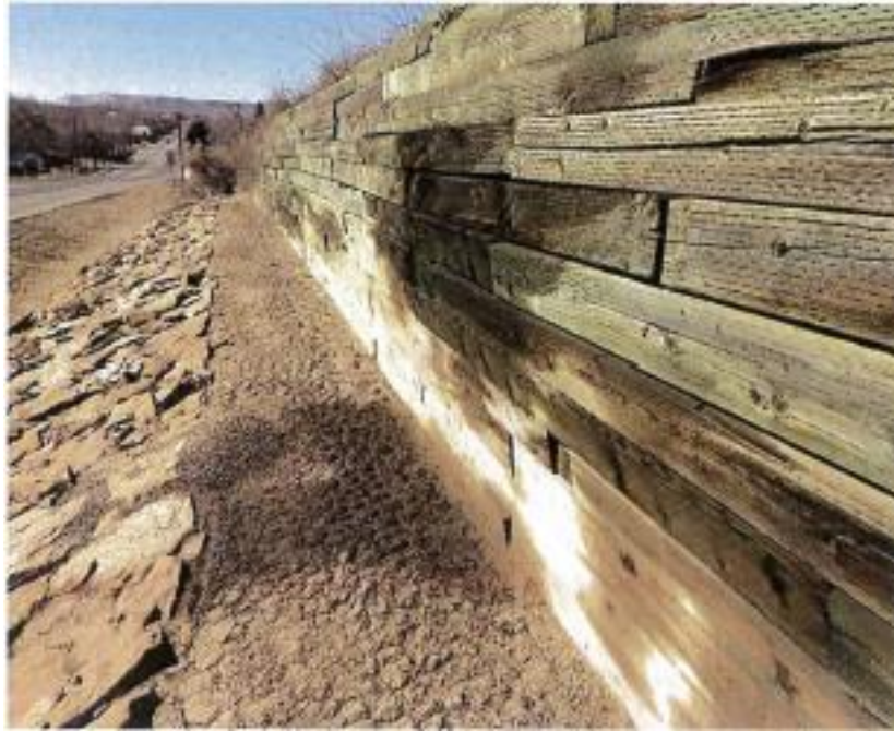
Figure 2. This treated timber retaining structure has been supporting the north side of Main Street/Hwy 64 for 30 years. The structure would be demolished and replaced with an attractive structure that complemented the final design of the south side retaining wall.
