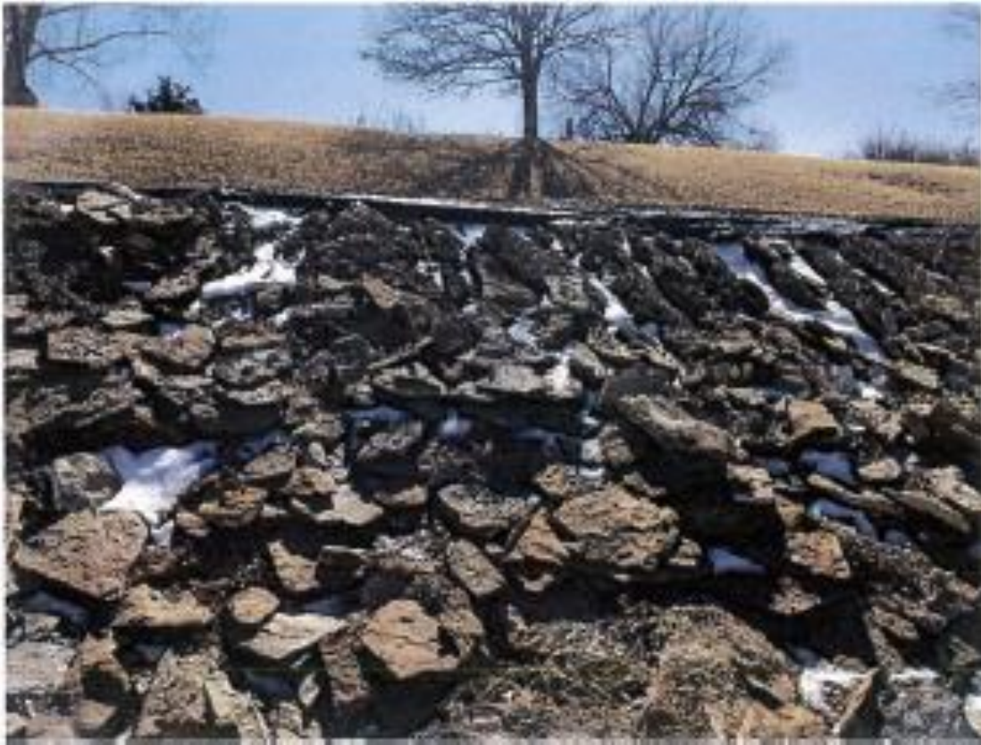
Figure 1. This shale and aggregate hillside continues for over 300' on the south side of Main St./Hwy 64. It was constructed in the late B0's in order to provide for stabilization of the soils and 10' wide bike/pedestrian path on top of this slope.
