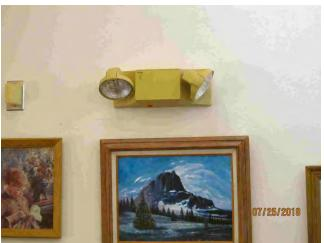
2018-2: White River Village – The emergency lighting unit should be repaired. It did not work when tested. It possibly needs a battery.
