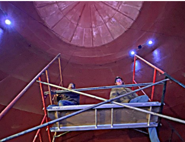
WCS employees John Sawsett and Justin Rusheron the scaffolding they constructed inside the TANK
