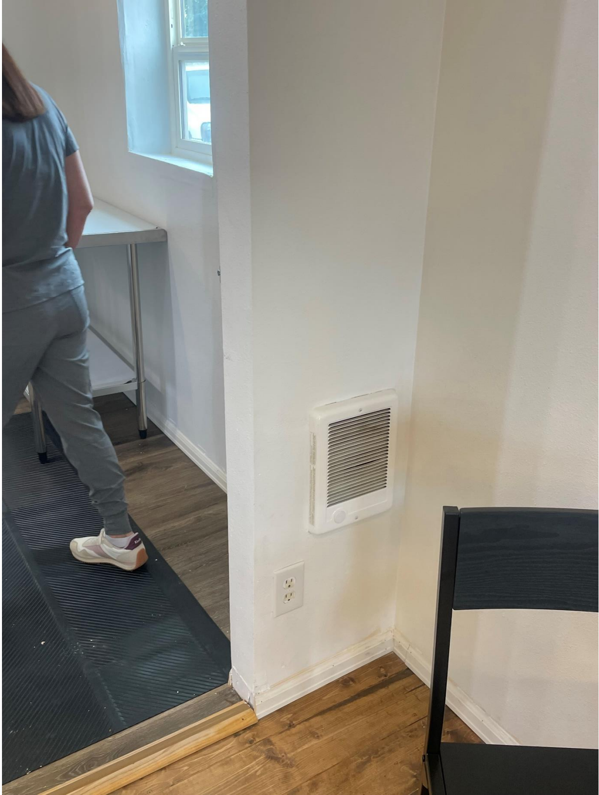
Figure 8. Wall heater in front section of bldg.
