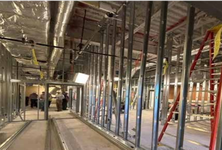
Steel walls in place, this view shows a storage room, to the left is the operating room and to the right clean sterile rooms.
